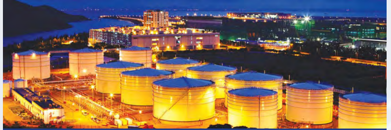
Storage Tank Inspections
