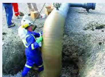
Pipeline wrapping Above & below ground
